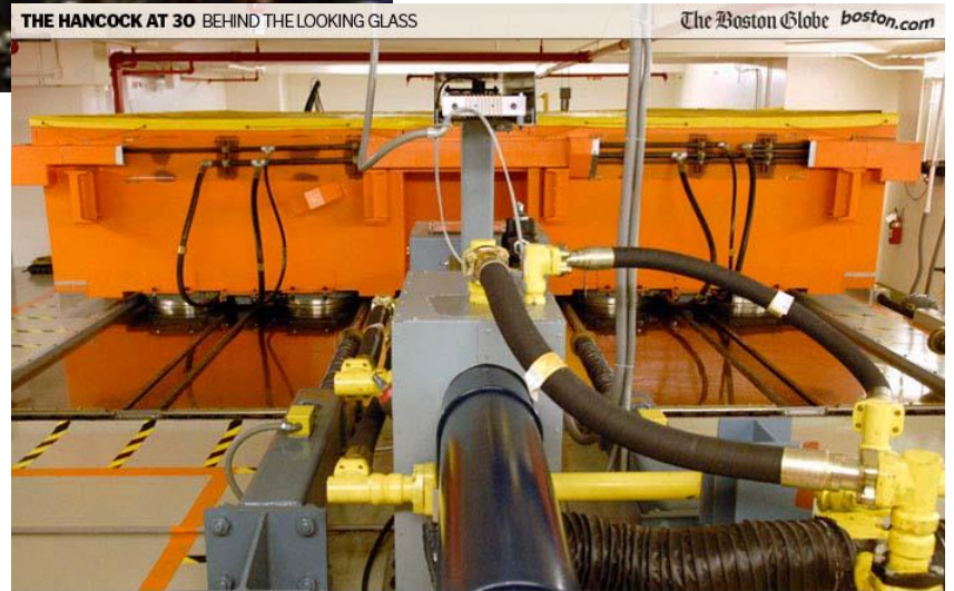
The tuned mass dampers
