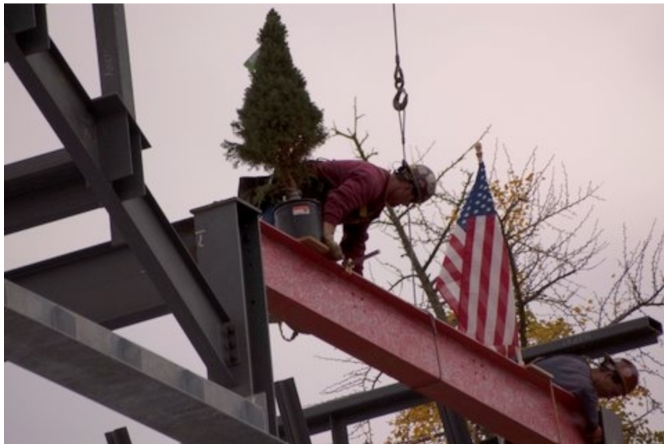
Figure 3.1: Installing the Student Beam in Muhlenberg's Seegers Union extension
